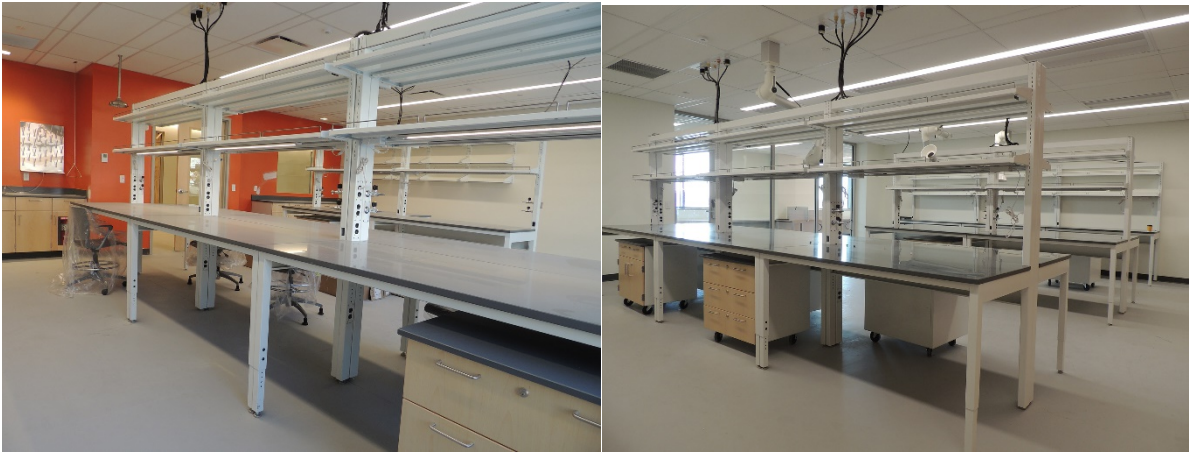
Internal Labs under construction
