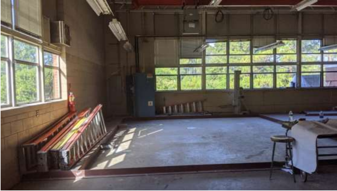
Southern CORE Foundry Lab Construction
